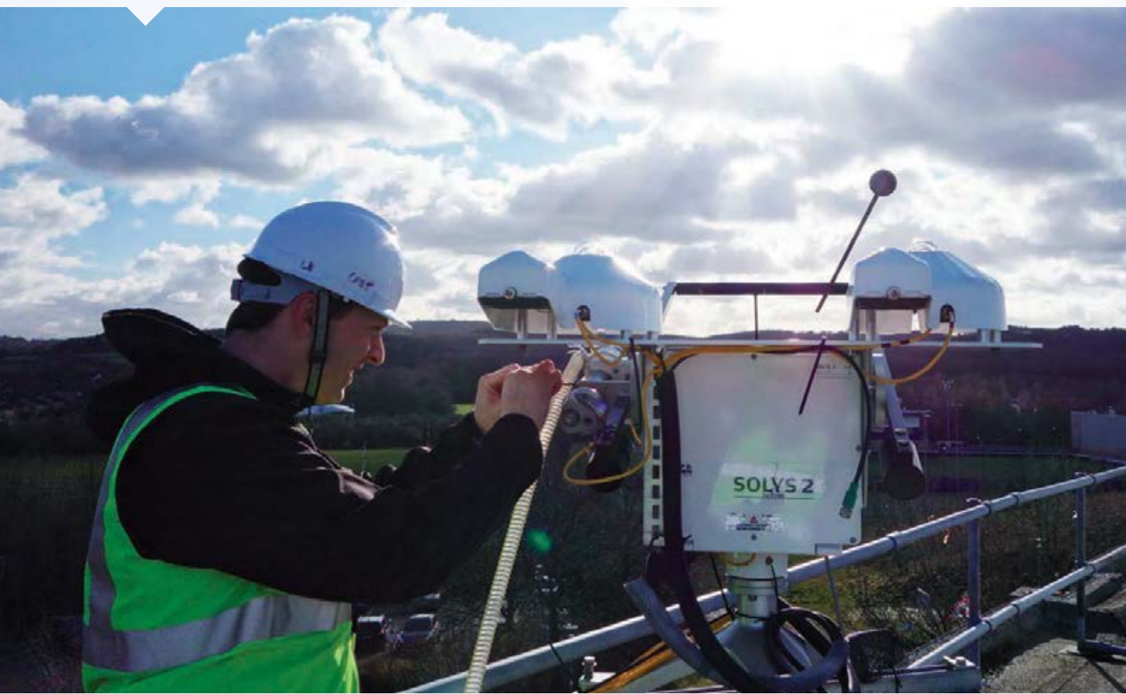
AirShield DNI installed and almost ready to operate
